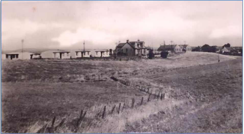
The prefabs at Park Street. See the article inside.
